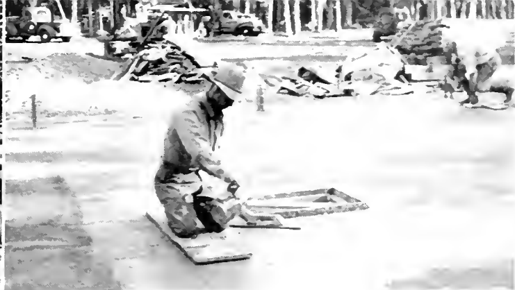
Finishing floor of truck shed on Sept. 26
